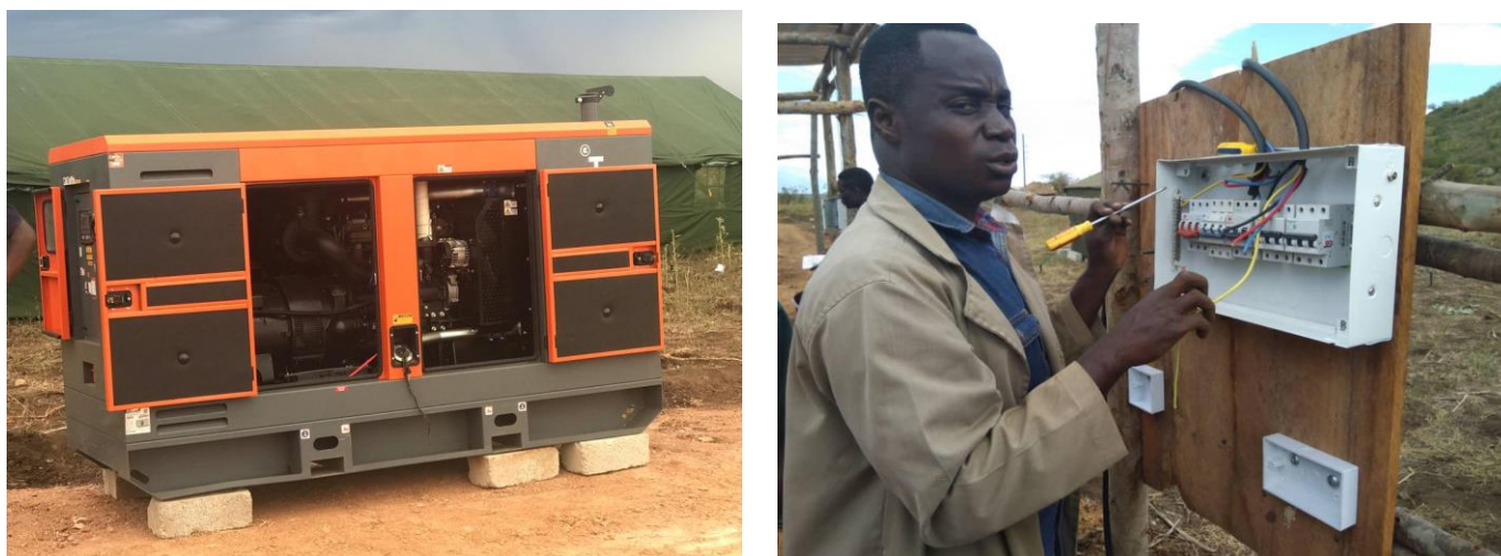
Fig 3. Generator for power supply to the block making machines connected.
