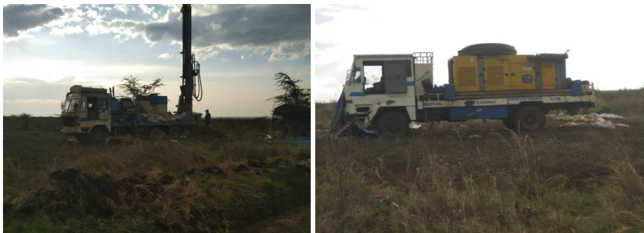
Fig 9. Drilling of powered water-production wells and boreholes on-going
